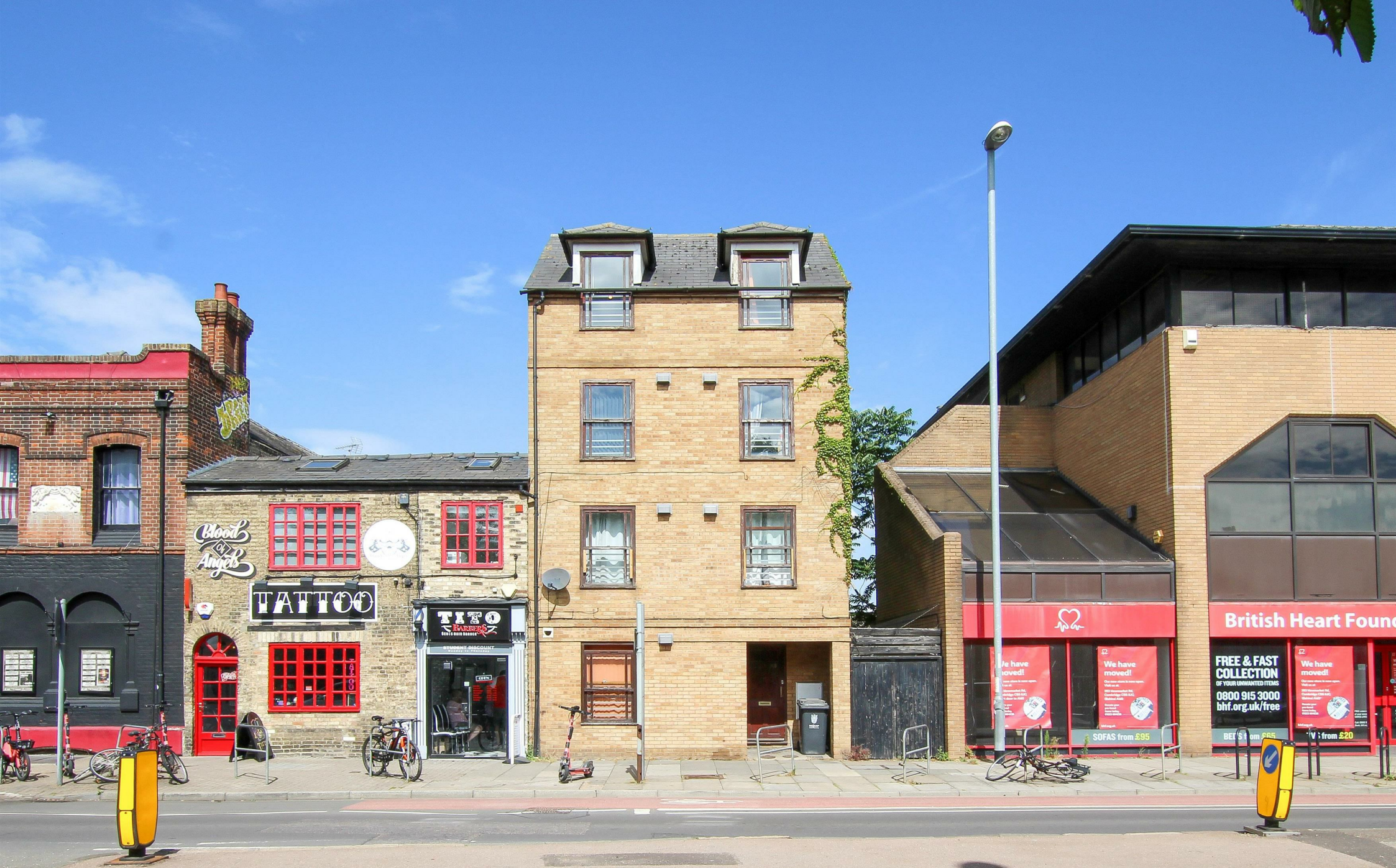
Room 1, East Road, Cambridge, CB1 1DB
